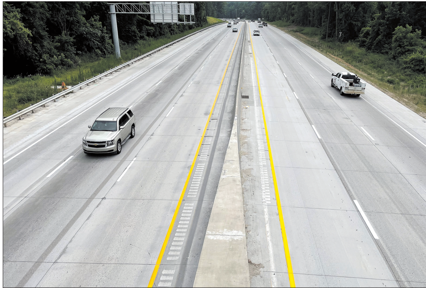
JOHN BURNS/RICHLAND CONSTRUCTION A
