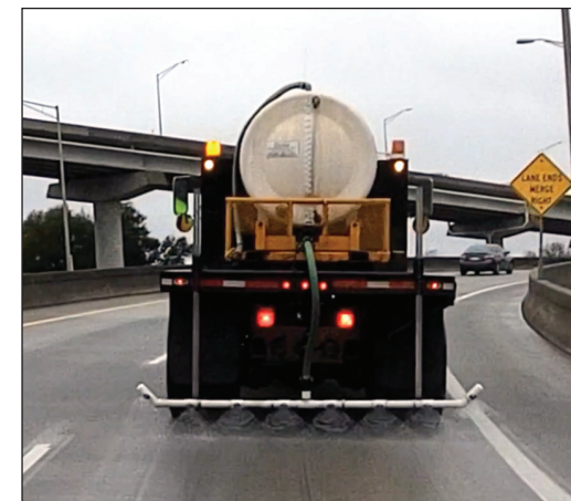
On Jan. 21, Charleston Maintenance pretreats I-26 ramps in Charleston. The back-to-back storms had crews working 24-hour shifts for almost three weeks.
