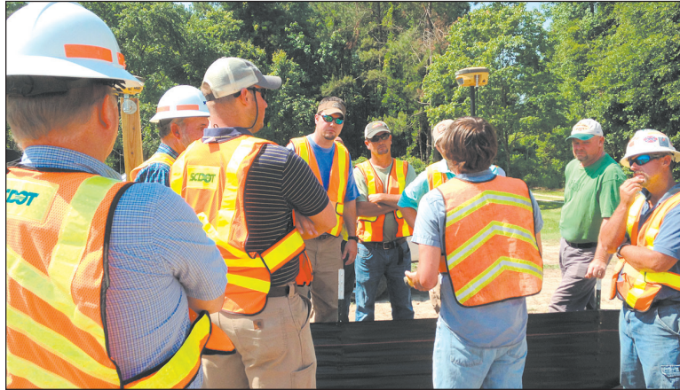
SCDOT District 5 construction crew took the 3D modeling for automated stakeout and inspection training at Florence US 378 construction site.
