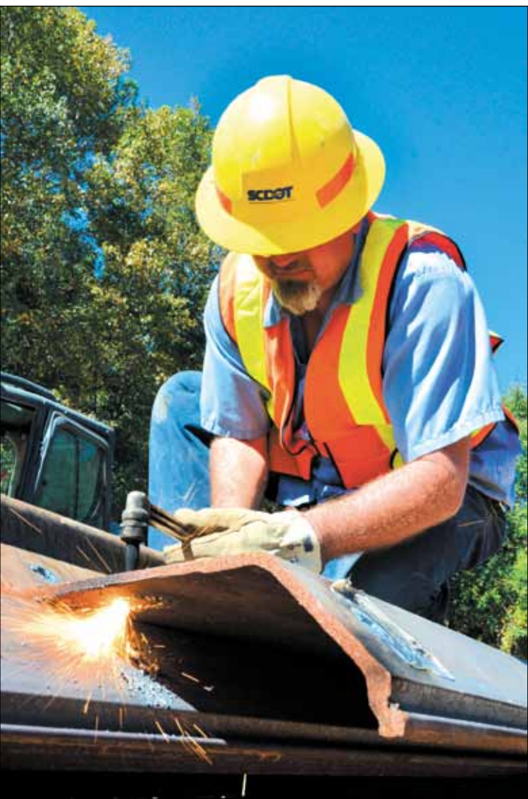
LEFT: Travis Floyd of Aiken Maintenance cuts sheets of pilings to size and cuts anchor holes into them as part of repairs to a washed-out bridge headwall on Fairfield Road in Richland County on Oct. 19.
