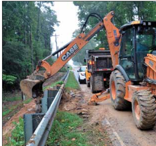
A crew from Lexington Maintenance repairs a washed-out shoulder along old Chapin Road in Lexington on Oct. 5.
