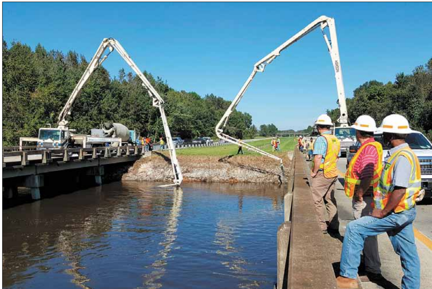
Scott McElveen, Michael Godwin and Wendell Jones of Clarendon Construction monitor concrete pouring underneath bridges along I-95 in Clarendon County on Sunday, Oct. 11. Six concrete pump trucks from United Contractors and SCDOT crews worked around the clock, seven days a week to shore up bridge pilings affected by flooding along the heavily traveled interstate.
