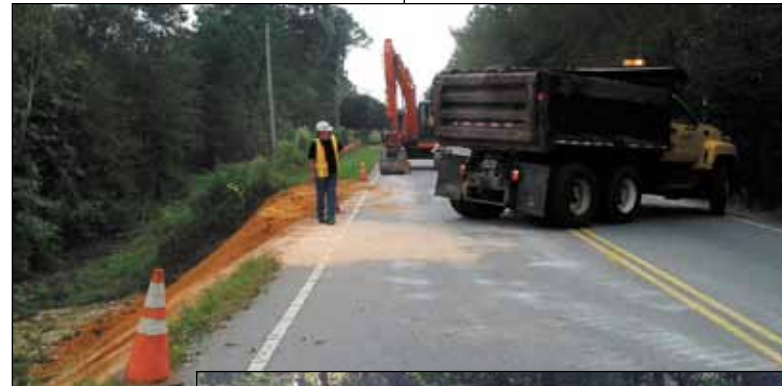
RIGHT: Workers from Fairfield and York Maintenance repair damaged bridge approach on Estes Lane in Fairfield County.
