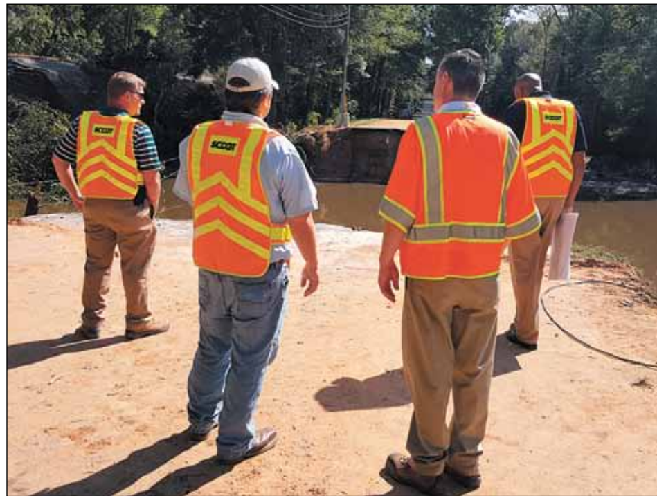
SCDOT District 1 engineers Paul Miller and Chris Kelly, District 1 Engineering Administrator Bryan Jones and Richland Maintenance Engineer Tony Magwood inspect damaged areas to decide the best course of action for repairs. On Oct. 8, they inspected the devastation of a washed-out bridge over Cedar Creek on Congaree Road.
