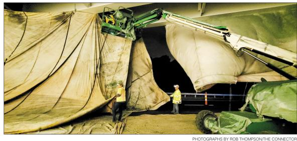
Before painting the steel bridge girders underneath, crews enclosed the area, including the roadway below it, with tarps to prevent overspray of green paint on the roadway and columns.
