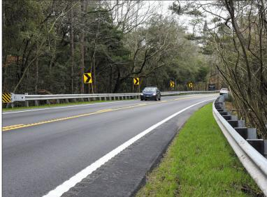
Featuring 11-foot wide lanes and 3-foot wide paved shoulders, center line and edge line rumble strips and updated guardrails and signage, this Rural Road Safety Program project makes this section of S.C. 61 much safer for the traveling public.
