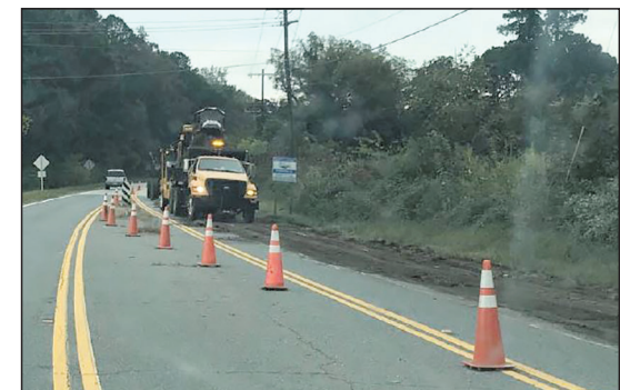
Crews do shoulder regrading in Chester County.
