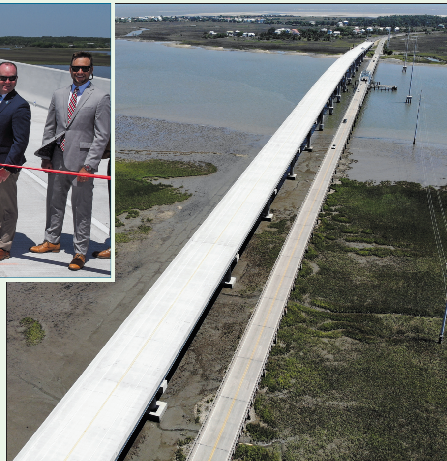
The new bridge is 3,350 feet long and rises 75 feet above the river. It will replace the old Sea Island Parkway swing span.
