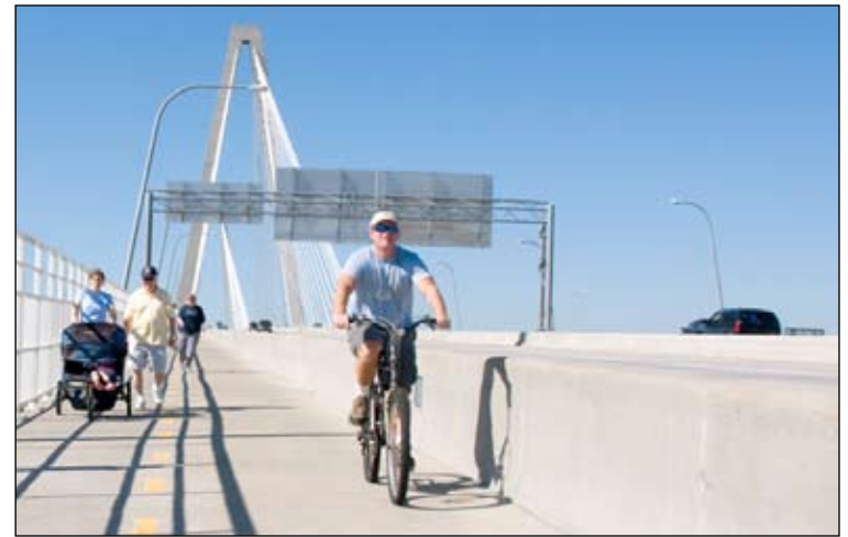
The pedestrian/bicycle path on the Cooper River Bridge in Charleston is popular with the public.
