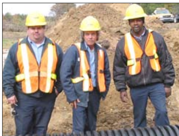
Driveway Crew is, left to right: Wesley McInville, Woody Moser and Jeffery Stroud install a driveway on US 321 in Chester
