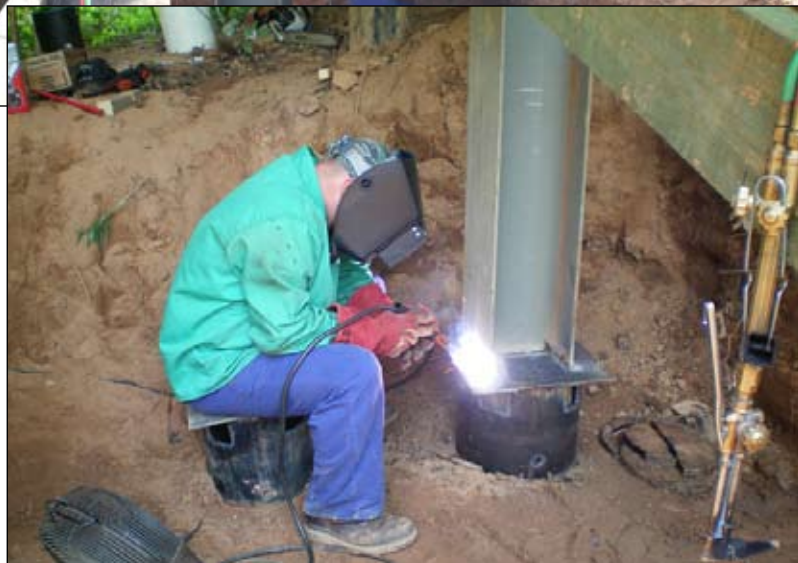
Craig Kyle, of Pickens Maintenance, is welding a new I-beam support under the bridge at SC 135 and Glenwood Road.
