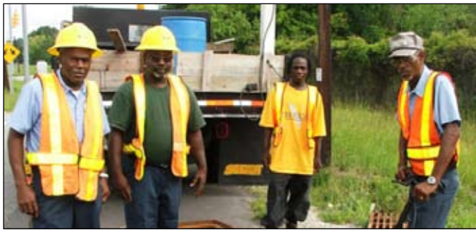
The driveway/concrete crew is: Leon Adams, John Gethers, Dennis Maxwell and Kenneth Bradley.
