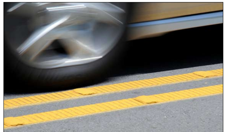
New 'Profile Thermoplastic Edge Lines' are shown above and at right. The ribbed surface helps warn drivers if they wander out of travel lanes.
