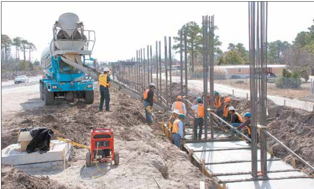
ABOVE: Crews construct a noise barrier wall along the North Myrtle Beach Connector project.
