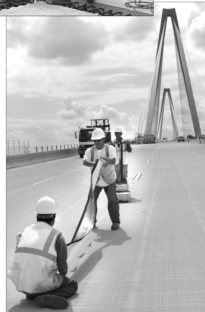
BELOW: Workers place striping down on the northbound lanes of the new bridge.
