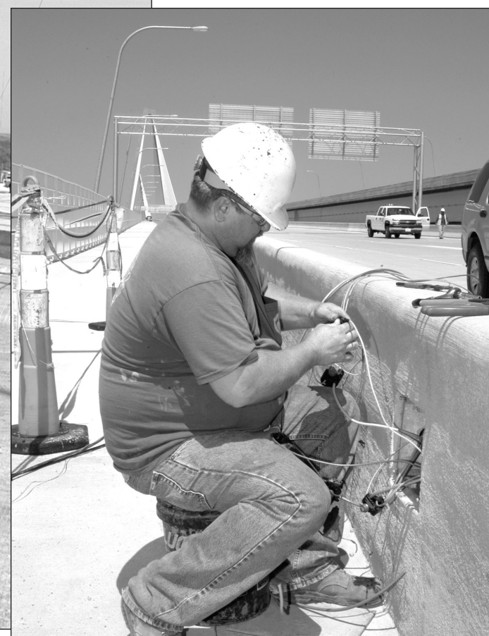
An electrician connects wires to install lighting on the bridge deck.
