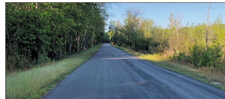
AFTER: The finished project replaced pipes, moved utilities and put up barriers to prevent beaver damage.
