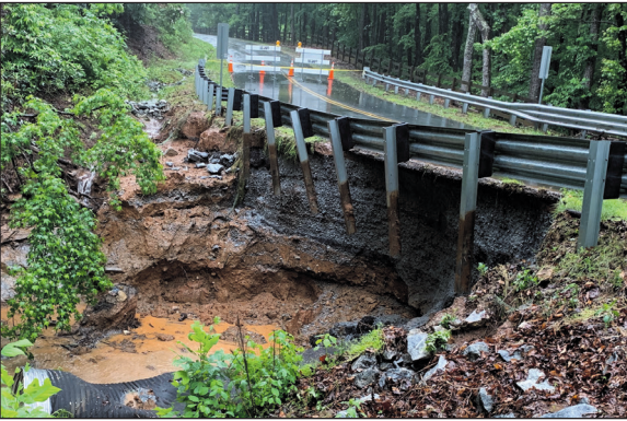
BEFORE: Dug Hill Road
