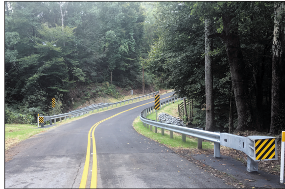
AFTER: Dug Hill Road
