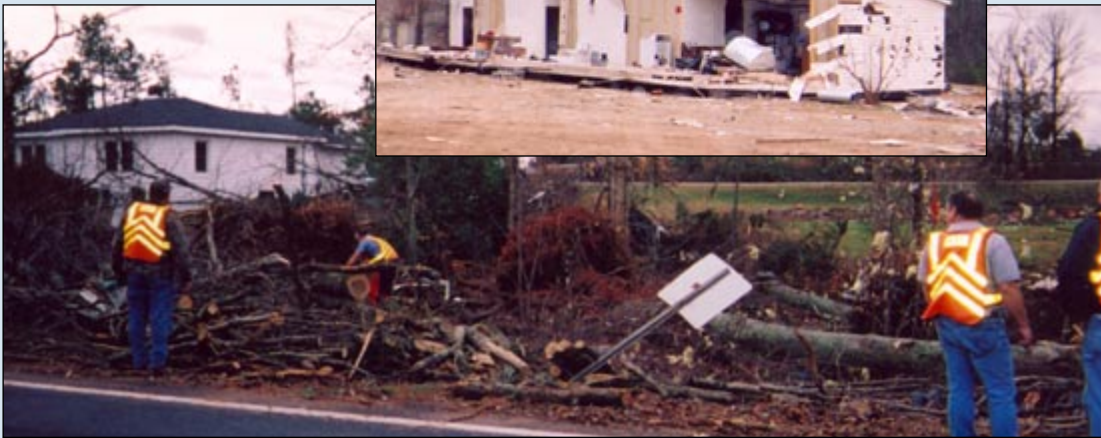
PHOTOGRAPHS BY RUDY KEETER/GREENWOOD MAINTENANCE Laurens Maintenance employees clear debris from a roadway after a tornado hit Laurens County. Above, one of the homes that was totally destroyed by the tornado.
