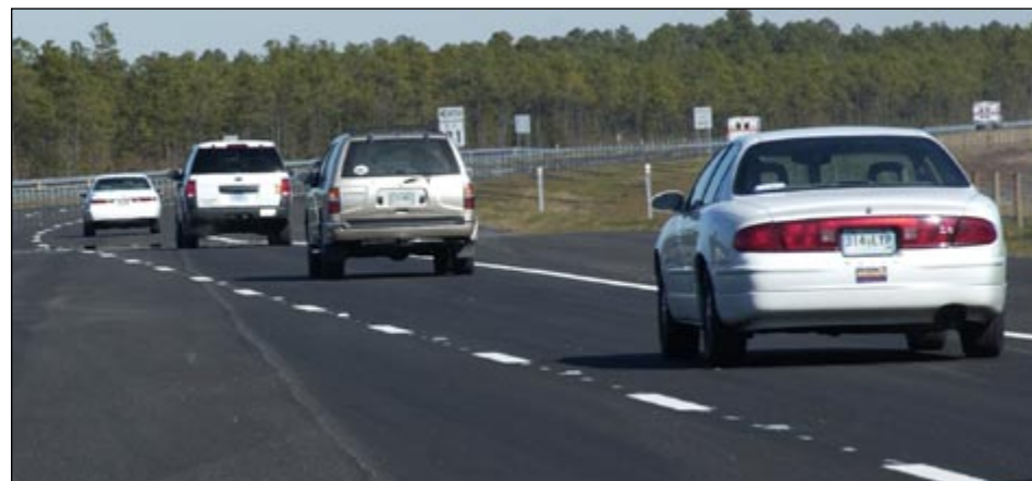
Motorists enjoy their first drive on the new section of the Carolina Bays Parkway.
